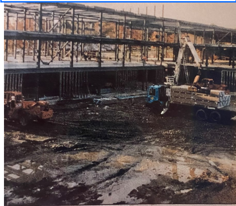
MIDDLE SCHOOL ADDITION
